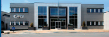
Pulaski Electric System Pulaski, Tennessee
